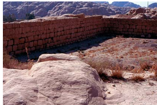
Water Management in Petra. Fig. 2 The Zurraba (al Birka) reservoir.
